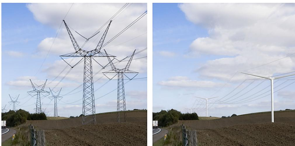
Figure 1. Traditional Steel Lattice Power Pylon (left) compared to a Composite Power Pylon (right)
