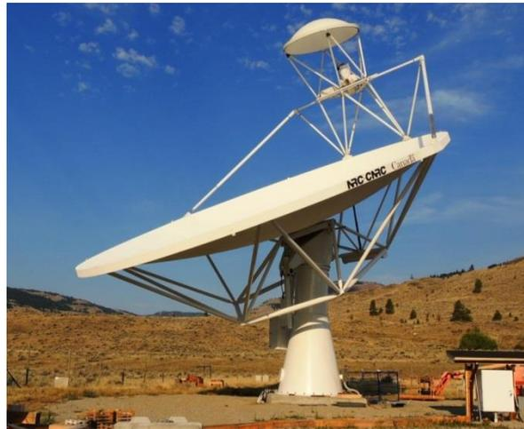
Figure 2: The DVA-1 single piece carbon composite radio telescope.
